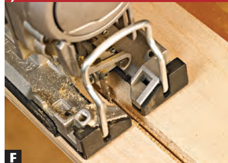
F After making a relief cut with a 1/4"-diameter router bit, we used a jigsaw to create clearance for the riving knife.
